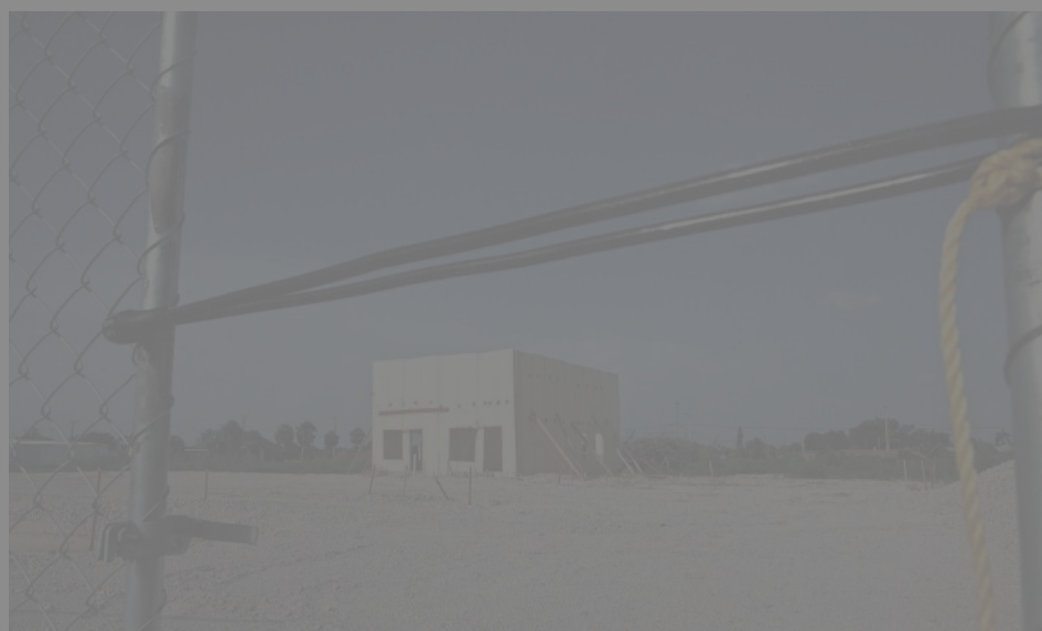
A makeshift structure stands on the property where the Towles Gardens apartment complex is supposed to be built. Work has stopped because of a dispute between the contractor and the developer. ANDREW WEST/THE NEWS-PRESS
